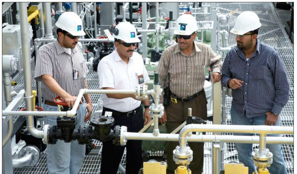
From left, plant console controller Ibrahim M. Shahrani, Rashid M. Shammari and supervising operators Aref S. Nehayan and Abdullah A. BuHaimed find one of the more than 60 flaws on the safety simulator skid at Abqaiq Plants. The skid gives new operators a chance to get familiar with possible safety hazards and plant veterans a chance to refresh their knowledge.
